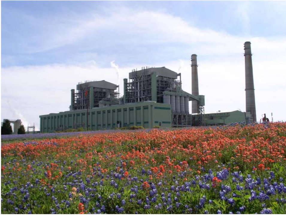
NRG Texas's Limestone Power Plant in Jewett, Texas
