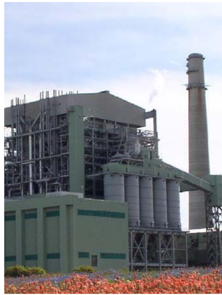
NRG's Limestone Power Plant
