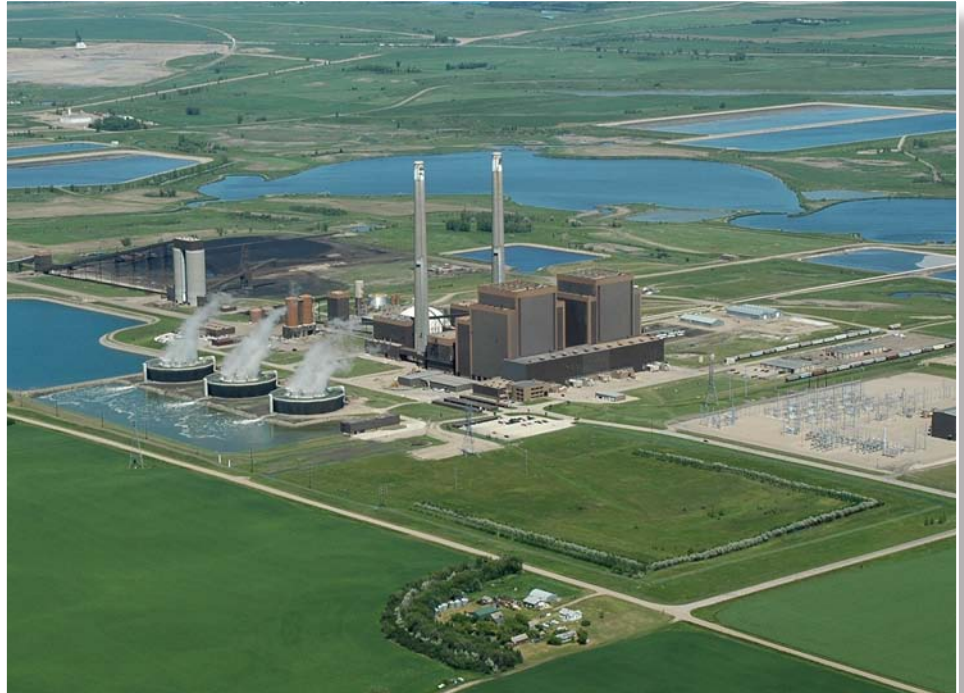
Aerial view of Great River Energy's Coal Creek Station lignite power plant
