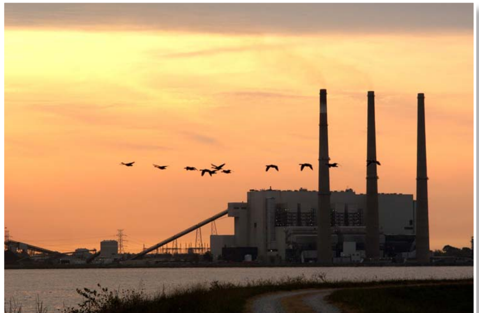
Dynegy Midwest Generation's Baldwin Energy Complex
